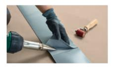
**12. Hot-air welding**Using hot air and pressure weld the tape joins with an overlap of at least 5 cm.
