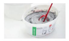
**4. Mixing of the mortar**Stir comp. A and comp. B together and put the mixture into a clean bucket. Then stir the mixture for a second time.
