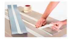
**3. Masking off the surface**Mask off the expansion area on the subfloor and on the tape. Mask off at the margin, the grout should overlap the building component by at least 1 cm.
