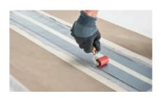
**7. Laying and pressing**Lay out the ASO-Tape and press it on-with a suitable tool.
