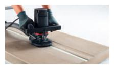
**1. Flooring preparation**Prepare the cleaned, weight bearing underfloor by mechanical means.
